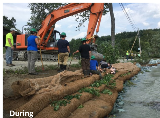
NSECC Training Day for bioengineering methods. Encapsulated soil lifts reestablish a gently sloped shore along Cedar Mountain Road on Lake Bomoseen, allowing native plants to root and stabilize the bank and road edge, while filtering and treating runoff before it enters the lake.
