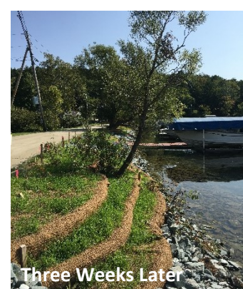
NSECC Training Day for bioengineering methods. Encapsulated soil lifts reestablish a gently sloped shore along Cedar Mountain Road on Lake Bomoseen, allowing native plants to root and stabilize the bank and road edge, while filtering and treating runoff before it enters the lake.
