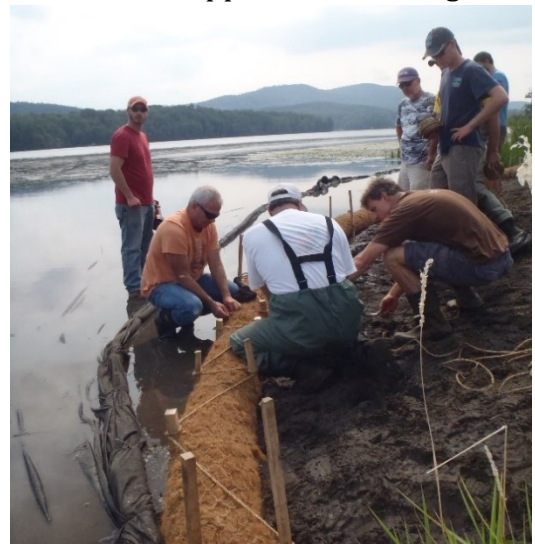
VT Agency of Natural Resources staff get trained in bioengineering methods in 2015 to install fiber coir rolls to stabilize an eroding shore at the Lake Iroquois Fish and Wildlife Access Area in Williston
